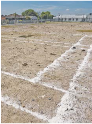
Square and fair: Outlines for construction work on one of the sites for the Elsie's River infill housing project. The project will eventually be home to over 700 qualifying beneficiaries, all selected and assessed fairly according to the City's established procedure.
