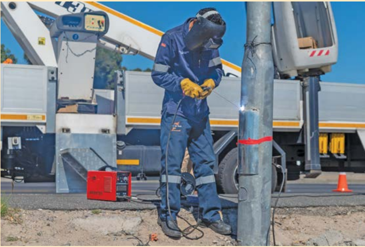
Keep calm and weld: The City remains committed to maintaining and repairing electricity infrastructure in Bishop Lavis and other vandalism-prone areas.
